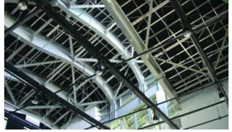
straight, universally oriented diagonal elements. While there are now several completed Gehry projects featuring this type of undulating metal roof surface, the performing arts center is the first design to expose the supporting structural framework at the building's interior.
