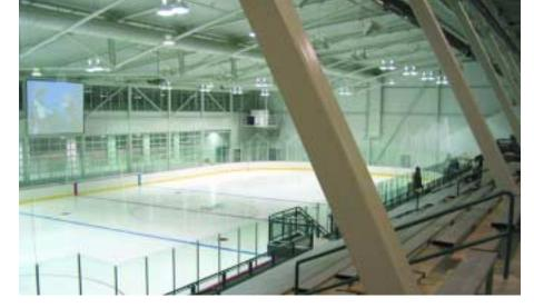
the roof trusses, and by keeping the lines of the trusses simple with a minimum number of members. An EPICORE roof-deck ceiling system spanning between trusses provided an appealing ceiling, supported the vertical loads, and provided the required diaphragm strength and stiffness.
